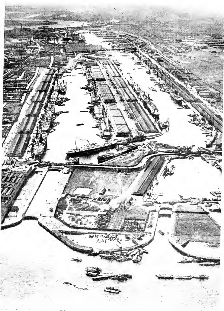
Aerofilms LONDON DOCKS. The Royal Victoria, Royal Albert, and King George V docks, which together form the largest sheet of enclosed dock water in the world (see diagram 62)
